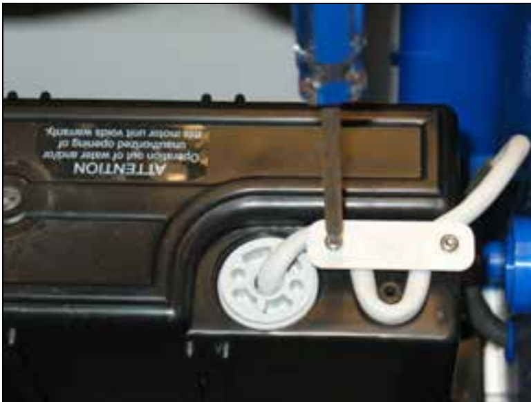
Remove strain relief cover plate.
