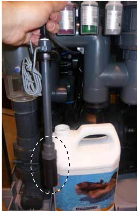
Figure 39: Particle filter
