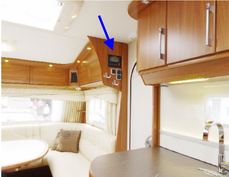
Left: The Control Panel mounted just next to the entrance in a caravan
