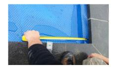
Align the clip and pre-pierce a hole in the blanket to allow for the placement of the clip screw. Attach the clip to the blanket and fasten.
