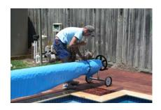
Cut the sun cover to the required size so it protects the full width of the blanket. Leave a 100mm overhang. To keep it in place, use the straps provided.
