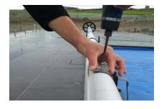
Adjust the straps so that each one has consistent tension when rolling the blanket onto the roller.
