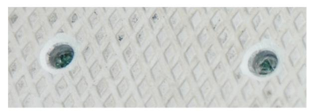
**Put 3M 5200 Adhesive in Holes and Base Location:** The 3M 5200 Marine Adhesive is a key structural part of any T-Top installation. Squirt 5200 into each hole and be sure it is filled with 5200. Then add a smooth layer about 1/16" thick between the four holes. The majority of the strength comes from the screws being bonded to the hole and the base being bonded to the deck adds additional strength. This should look like the image below.
