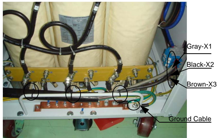
Figure 6 Input Power Cable Connections
