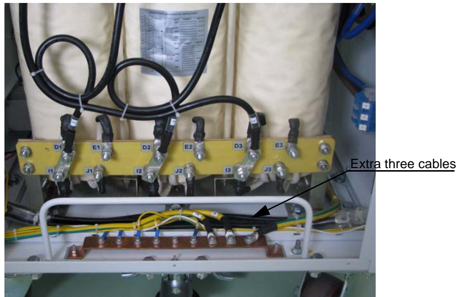
Figure 8 Position of extra three jumper cables
