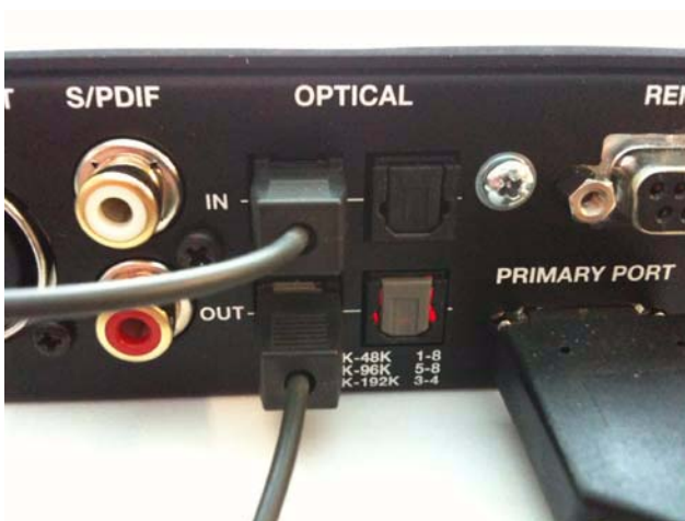
Figure 1. Optical loop back connections
