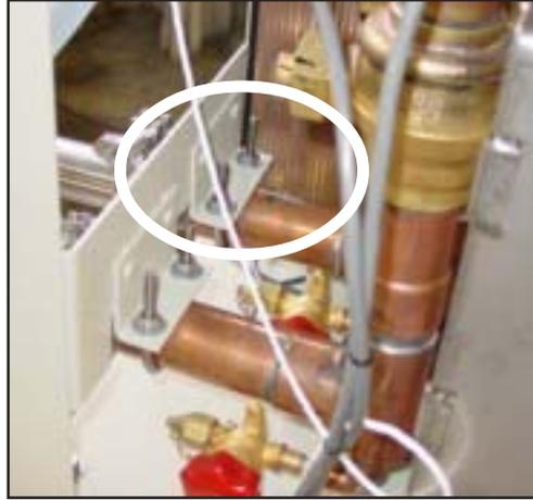
7. Undo the sanitary fitting at the heat exchanger.
