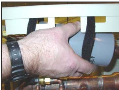
5. Install a new dryer assembly. Secure the Velcro straps first to prevent bending the lines.
