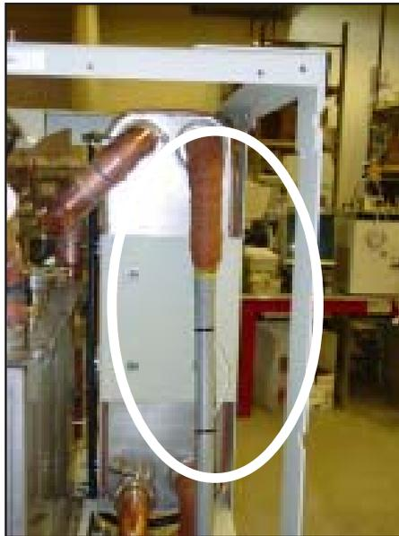
5. Attach new sensor with hose clamp.
