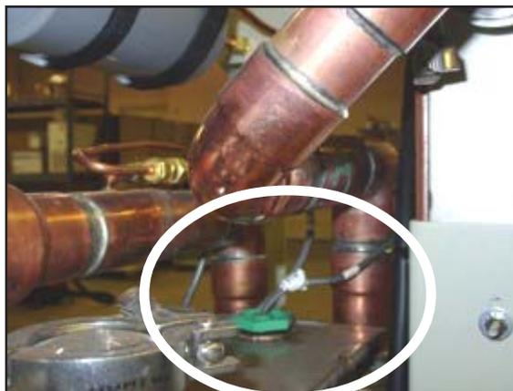
6. Once the unit is restarted check for leaks.
