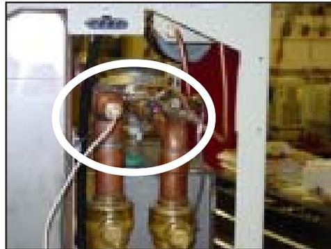
5. Use the 1/2" and 9/16" wrenches to disconnect the two process flow lines.
