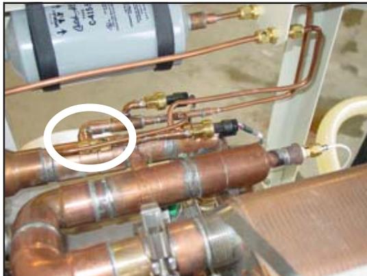
6. Undo the u-bolts securing the line to the unit.
