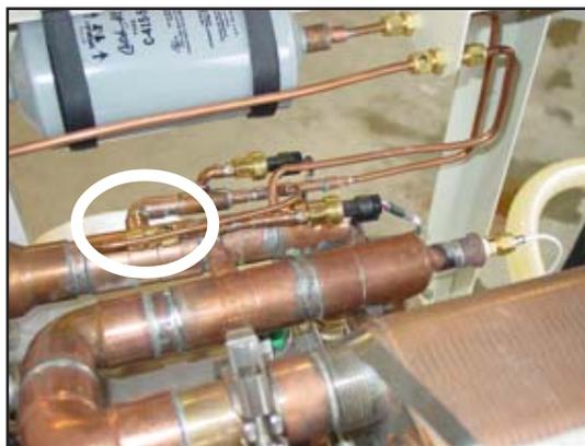
5. Use the 1/2" wrench to disconnect the process lines from the dryer.
