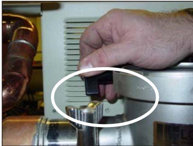
3. Remove the clamp. Note how the "T" is locked into position on the clamp.
