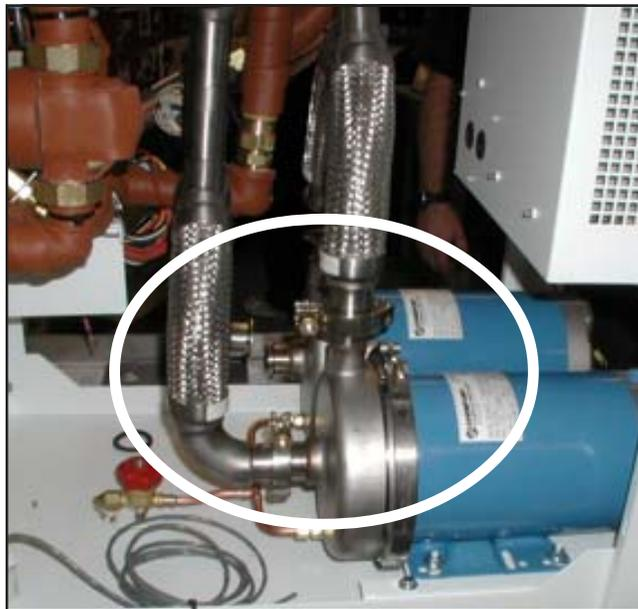
4. Using a 11/16" wrench, remove the fitting from the pump's drain line.
