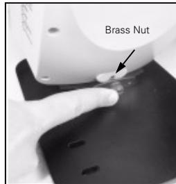
3. Tighten the integral screw until snug. Do not over-tighten. Verify the Spot Vital is fastened securely to the transformer mounting plate.
