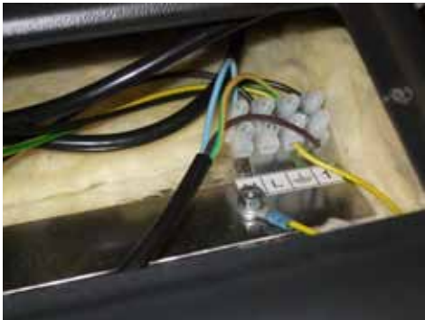
Connect the power supply to the screw terminals L, N, and PE.
