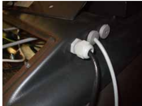
The burner's supply cable is installed from the factory. Install the BeQuem burner's sensor cable in the panel.
