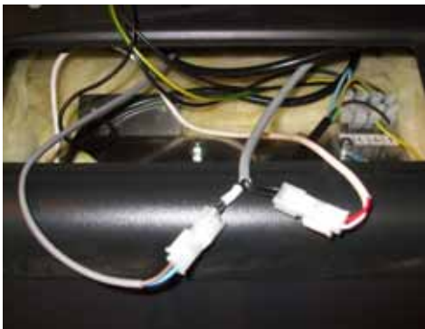
Connect cables to the smoke gas sensor (marked with white identification) and boiler sensor.
