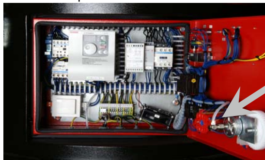
Fig. 9-2: Maintenance of the pressure annunciator unit
