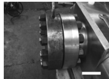
A finished flange should appear as shown.
