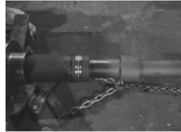
The finish weld should appear similar to the one shown above.
