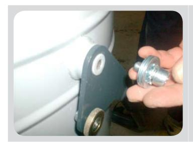
Unscrew the screws, then remove the normal washers and serrated washer.
