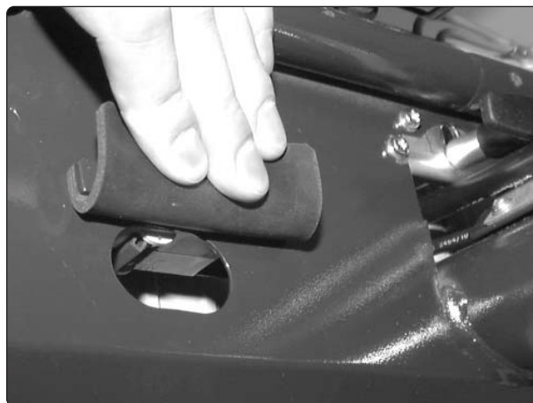
Main fuse/battery cut-out
