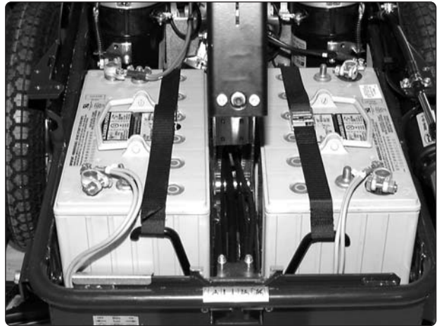
Cable laying at the batteries (seen from the front)
