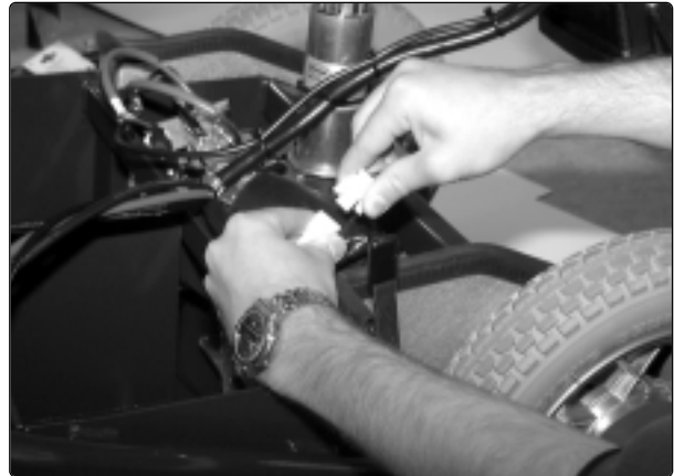
Electrical connection of the magnetic brake
