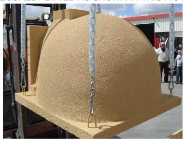
THE OVEN WEIGHTS APPROX. 1400 LBS. PLEASE ENSURE THAT ALL EQUIPMENT AND MATERIALS USED FOR LIFTING THE OVEN ARE RATED FOR LIFTING WEIGHTS ABOVE THAT OF THE OVEN. THIS INCLUDES CHAINS, STRAPS, HOOKS, PULLEYS, ENGINE HOISTS, AND ALL OTHER EQUIPMENT.
