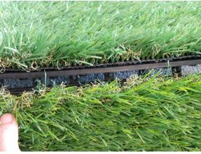
3. FOLLOWING THE SAME FIBRE DIRECTION, PLACE NEXT TILE ABOVE THE FIRST TILE WITH MALE INTERLOCKING CLIPS JOINING THE FEMALE INTERLOCKING CLIP OF THE FIRST TILE LAID. ONCE INTERLOCKING CLIPS ARE INLINE PRESS DOWN FIRMLY TO LOCK TILE.
