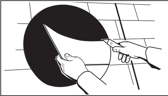
6. Remove the template and cut out the shingles inside of the circle.
