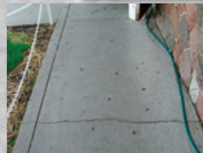
If you fail to properly design for shrinkage uncontrolled random cracks will occur
