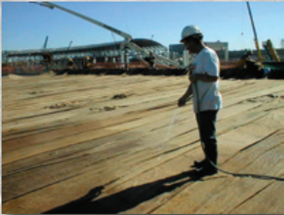
Proper concrete curing practices significantly reduce dusting problems
