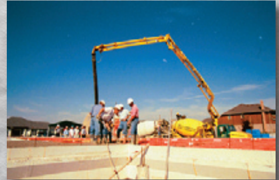
Concrete pumping on a residential radiant floor heating project
