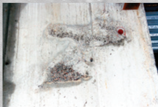
Honeycombing in a concrete column
