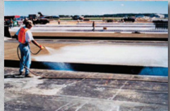
The proper application of a curing compound
