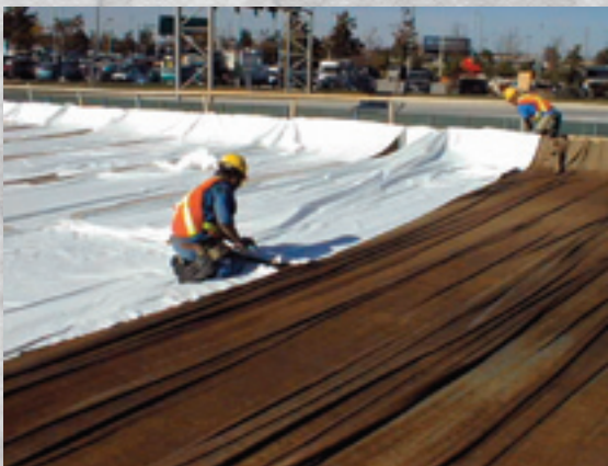
Proper concrete curing practices significantly reduce instances of concrete scaling
