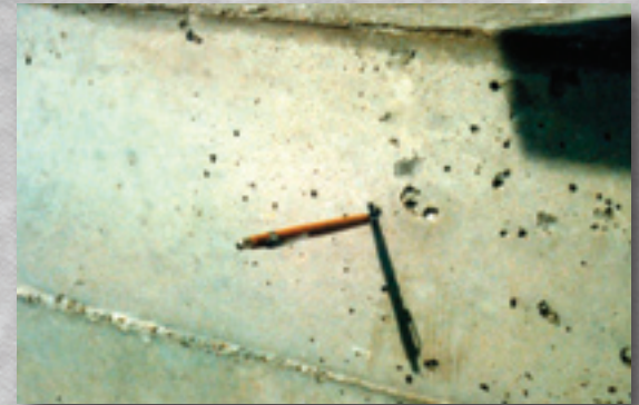
Bugholes on a plywood formed surface
