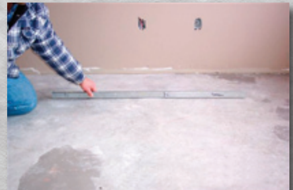
An example of a wavy concrete surface
