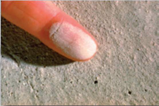
An example of a dusting concrete surface
