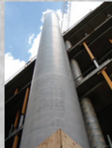
Bugholes on a plywood formed surface
