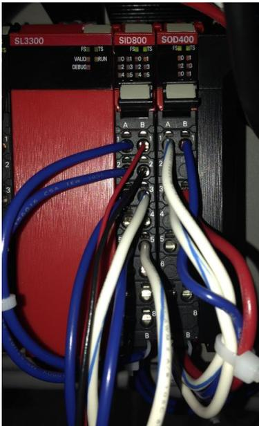
Image of NX CPU, SID800 input, SOH400 output.
