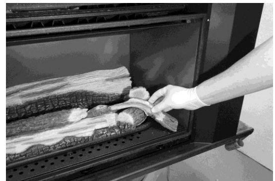
Figure 41: Decorative Log Installation
