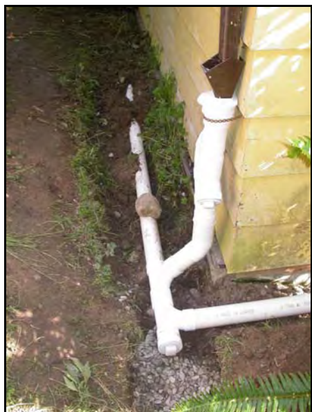
The 8" all-in-one debris pipe during construction and at completion
