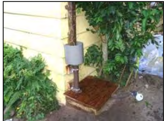
Leaf trap combined with 3" debris trap and pipe cleanout plug
