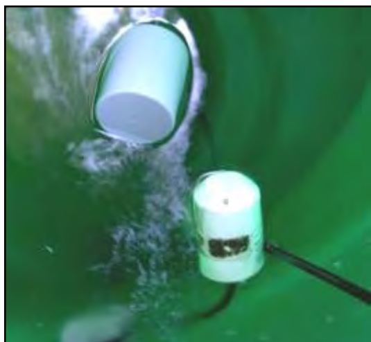
Float switches and cable weights
