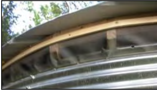
Screened venting at roof overhang
