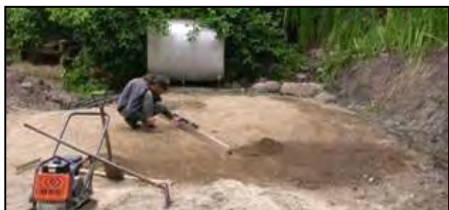
Removal of top layer of soil
