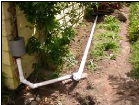
Leaf trap combined with 3" debris trap and pipe cleanout plug
