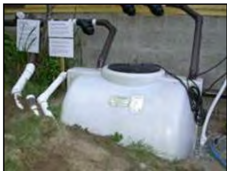
Tap and blue hose allows easy emptying of tank for cleaning.
