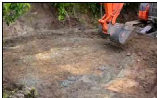
Removal of top layer of soil
