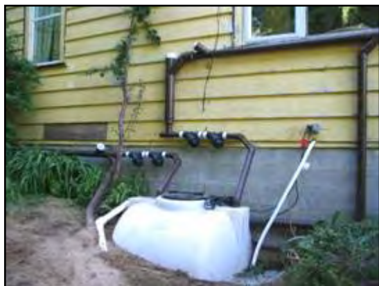
175 imp gal surge/pump tank showing water and electrical connections to house
