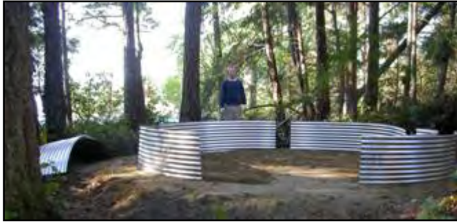
Starting the first ring of a bolt-in-place tank
