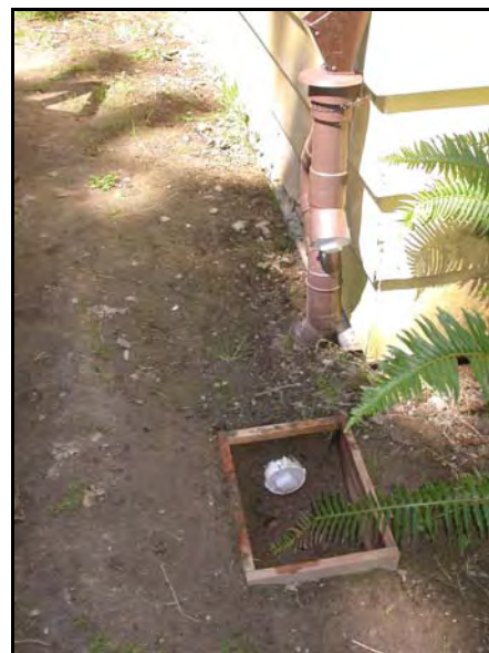
The 8" all-in-one debris pipe during construction and at completion
