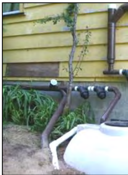
West side catchment piping, mesh screen filters and entry to surge/pump tank
