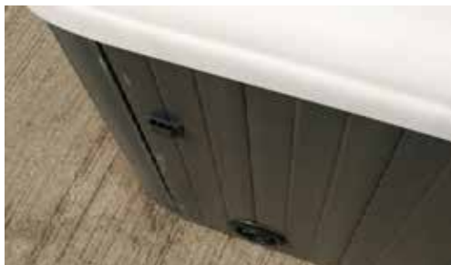
Ensure the drain valve is left open (i.e pushed in)
