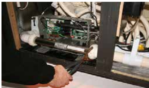
Disconnect the inlet and outlet union to the Control Pack
