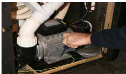
Remove the motors, pumps, electronics, and blowers and store them in a warm dry place
