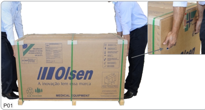
P01 1- Place the box next to the installation site. Use the existent handles for transportation.
