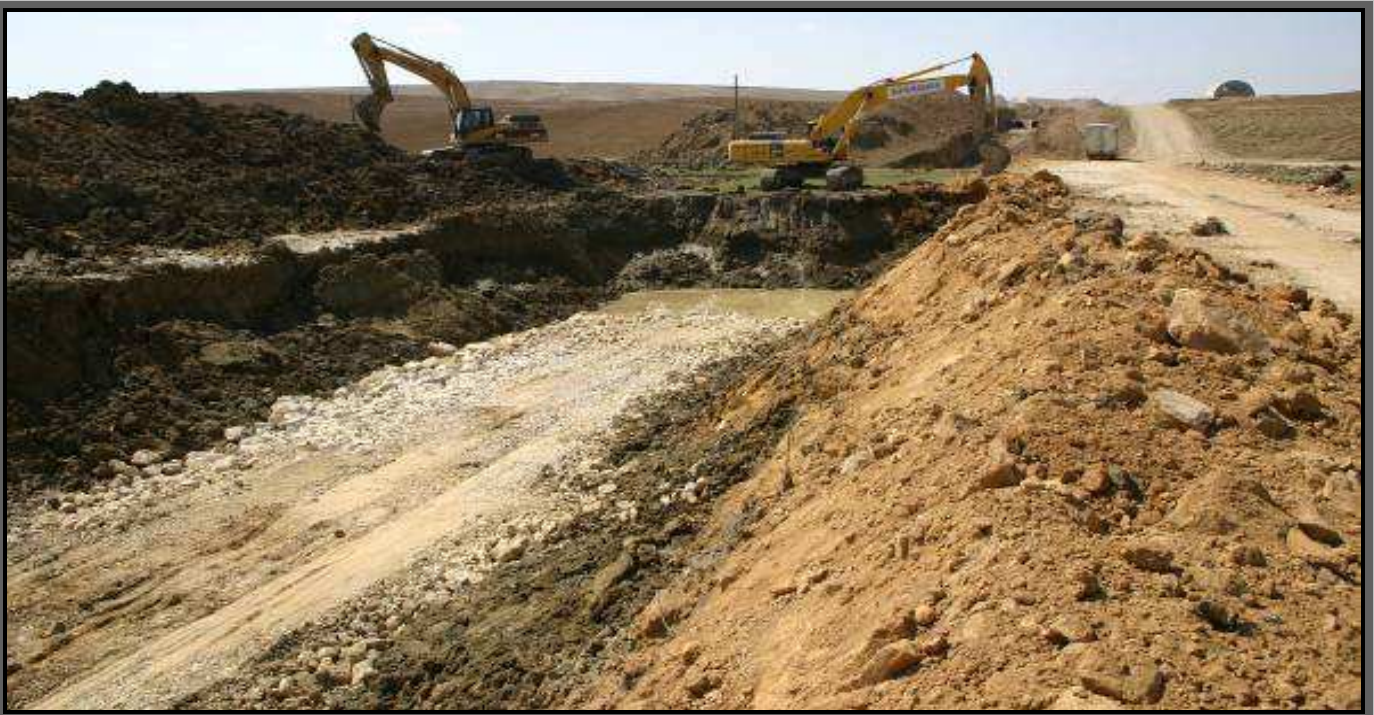
Trench ground stabilization works (Foundation)
