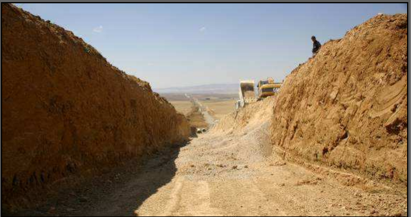
Bedding after ground stabilization
