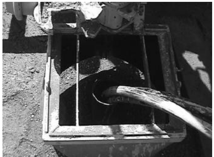
Inserting Plastic “U” tube in 4” Borehole
