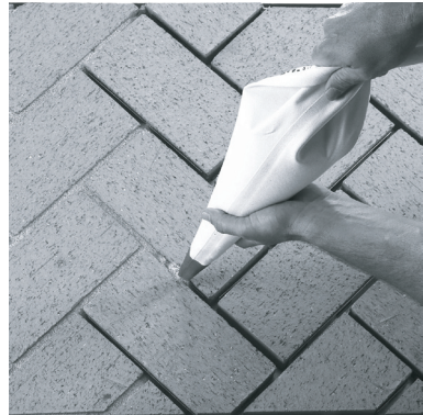
Figure 25 - Grouting Brick
