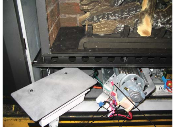
Resistor Con-nectors Fan Connectors Fan Ground Cable
