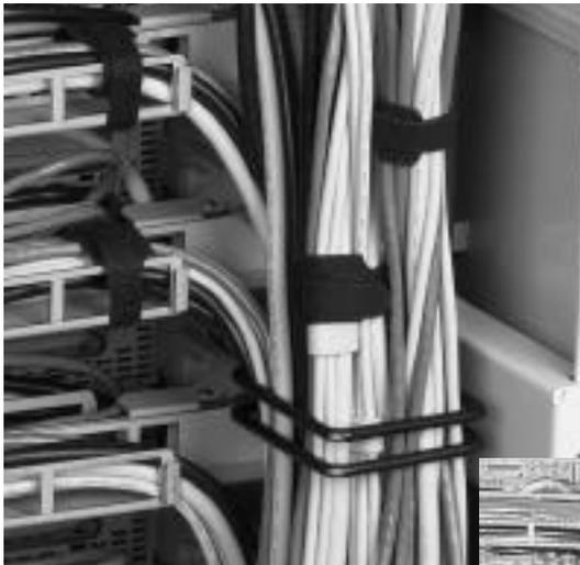
Systems are generally designed for specific requirements and will differ from each other. But when multiple servers are mounted in a rack, most KVM (or console switch), peripheral and LAN cables are routed down towards the floor and out through the cable opening. Power cords, however, are generally connected to the appropriate Power Distribution Unit (PDU) within the rack.
