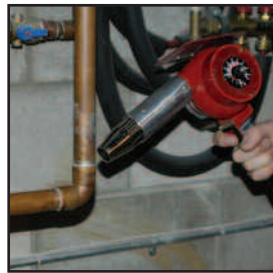
Solder Copper Pipe
