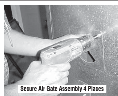
Figure 13 - Install Screws
