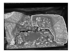
**Figure 8.9** Place the right log on the log shelf along the back of the firebox with the front of the log resting on the burner.
