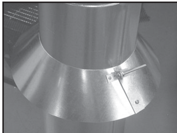
Figure 8.17 Assembling the Storm Collar Around the Pipe
