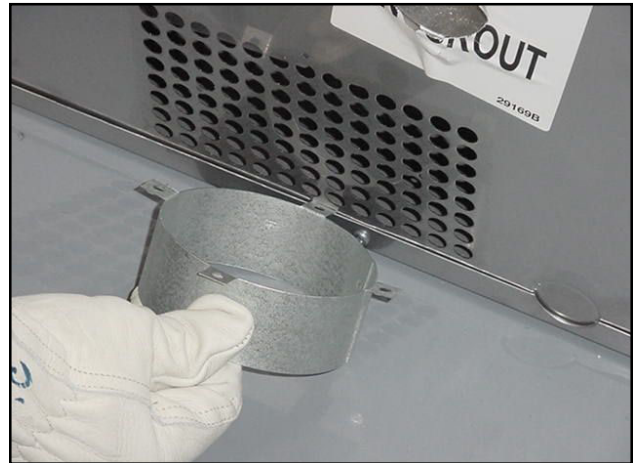
Figure 18 - Slide the Tabs
