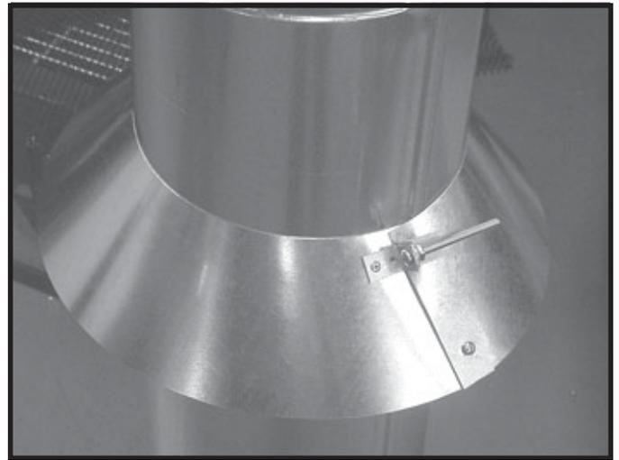
Figure 8.16 Assembling the Storm Collar Around the Pipe
