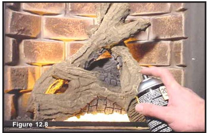
**STEP 6:** Turn on ember light/ember bed. Use high temperature black paint and lightly fog the clear rock.
