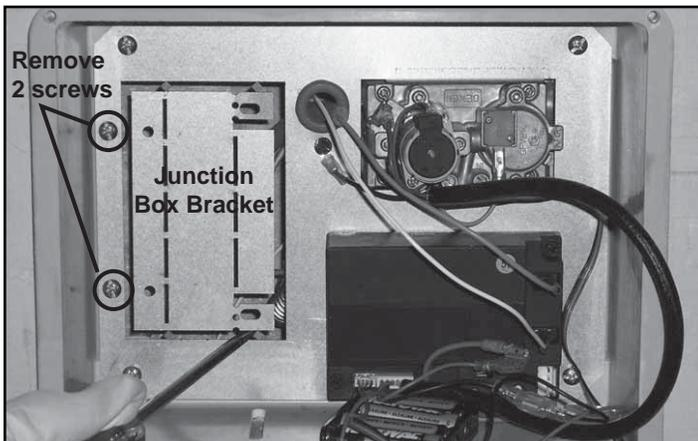
Figure 6.4 Remove Junction Box Bracket & Two Screws
