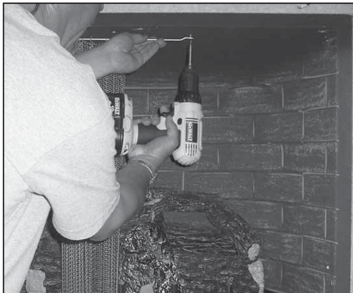
Figure 8.14 Fasten Screen Rod to Firebox Top
