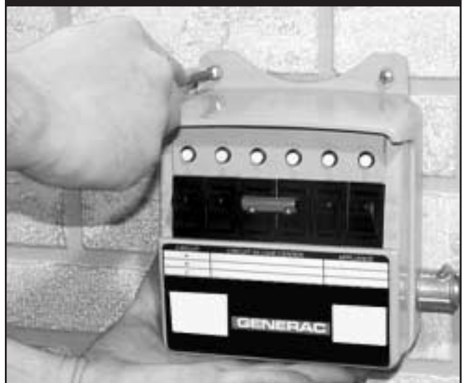
Figure 4 — Anchoring Load Manager™ Switch
