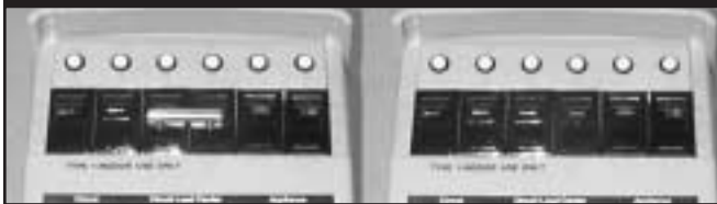
Handle Tie Installed
