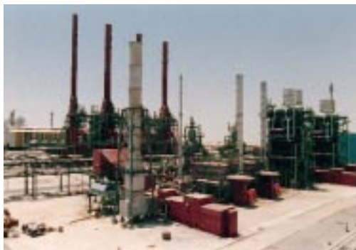
Rhourde Nouss - Algeria MS5001 - MS3001 Gas Turbines and 2BCL 406B Compressors
