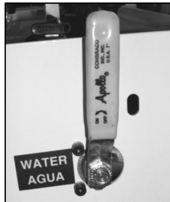
**Figure 17: Water Valve Assembly**
