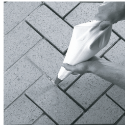
Figure 23 - Grouting Brick
