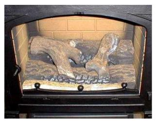
The base and front logs are fixed in position and should only need removing for servicing. The base log locates onto the burner and the front log is pushed to the extreme left hand side. Take the 2 loose logs\* and position them as shown onto the cut outs on the base log, taking care to locate them correctly to ensure clean combustion. No additional logs should be added to the fire.
