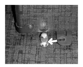
The piggy-backed amp can be rolled around on its casters by the amp head's handle, but **do not** try to pick the combo up by the amp head or its handle
