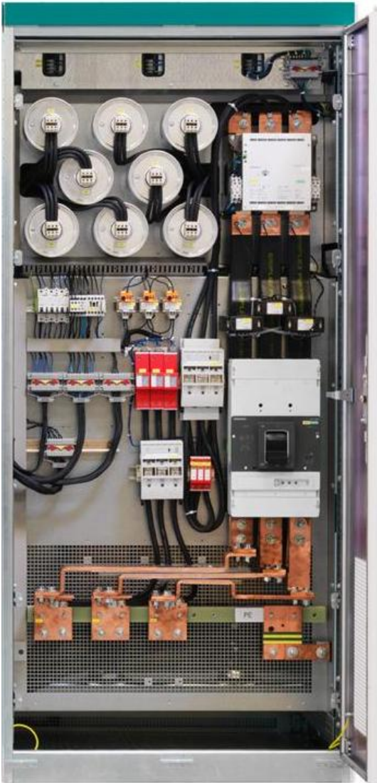
Figure 3-24 Armoire CA SINVERT 500 TL
