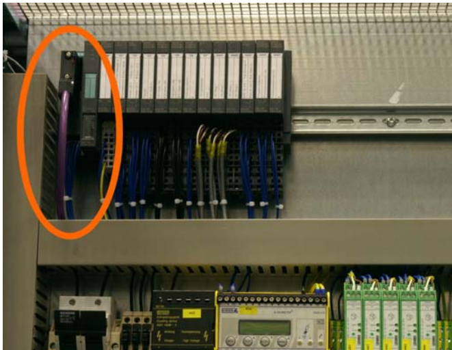
Figure 4-18 Connexion Profibus
