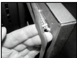
Picture F10: checking the fire door seal
