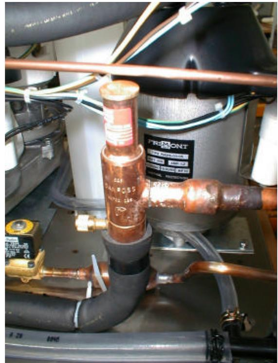
The refrigerant system is supplied completely sealed with two copper caps located on the flared nuts and pre-charged with a limited quantity of R404a.
