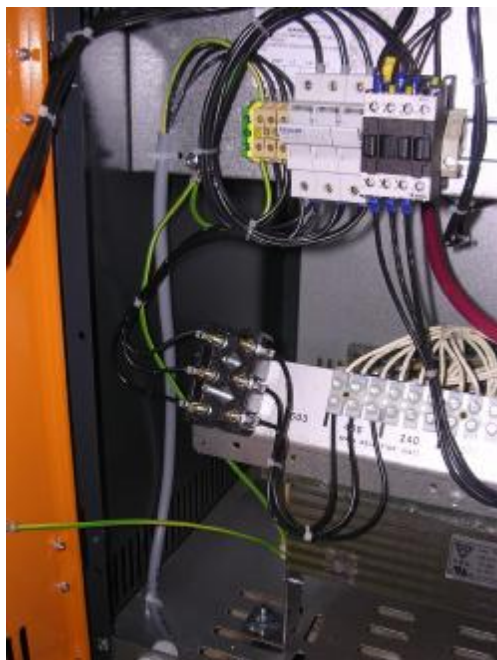
This Picture shows how mains connection to LP cabinets is performed
