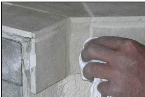
8. Quickly fill one portion of the seam line with the epoxy mixture. Remove the excess epoxy material from the seam line using a razor blade.
