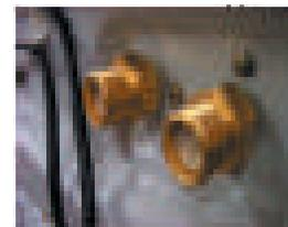
Brass Pressure Regulators installed on back of appliance.
