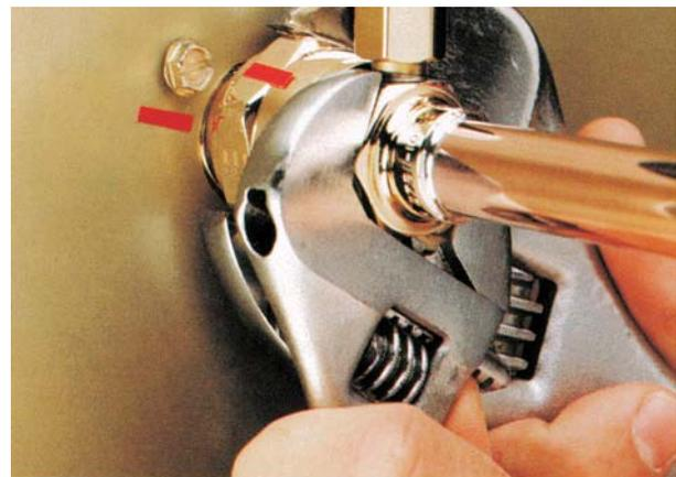
5. Use a marker or pen to mark a line on the coupling nut and unit panel. Then tighten the coupling nut an additional one-quarter turn. The line will show the amount that the nut turns. Do NOT over tighten.
