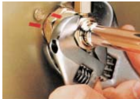
Rotate Swivel Nut \frac{1}{4} Turn More
