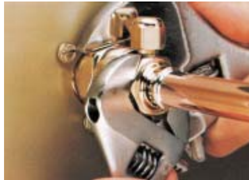
Tighten Swivel Nut
